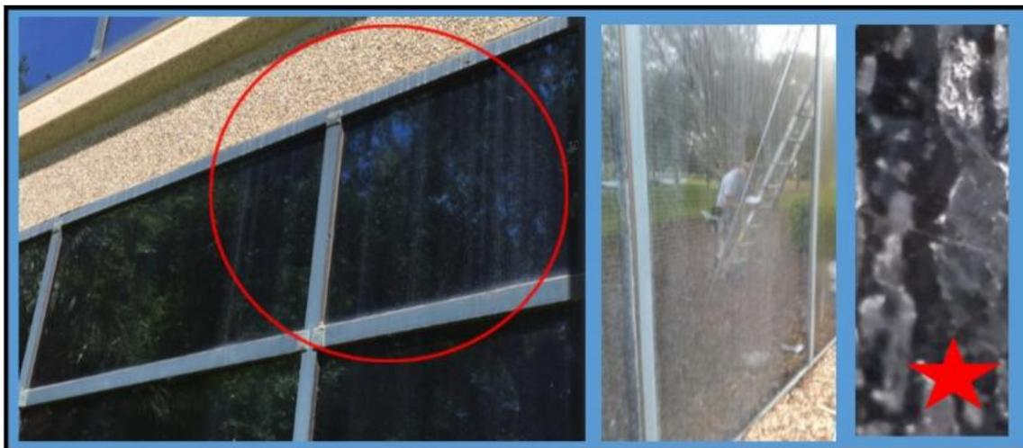
**\*\*Close-up view of EFFLORESCENCE STAINS on glass.**
